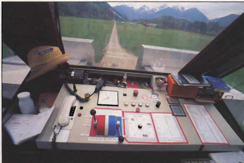
The control panel showing the view to the launch point over the backs of the motor-houses and winchdrum boxes.
